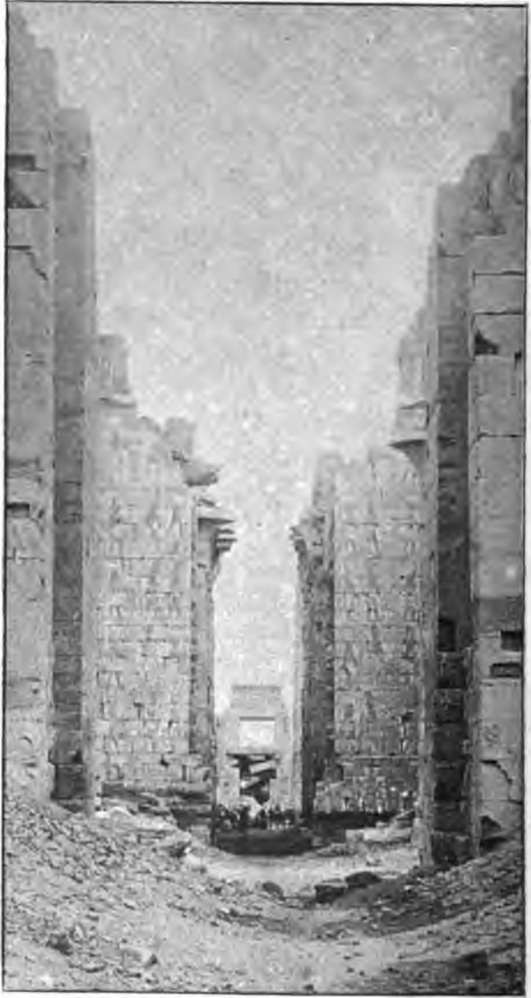
FIG. 12.—The axis of the Temple of Karnak, looking south-east, from outside the north-west pylon (from a photograph by the author).
